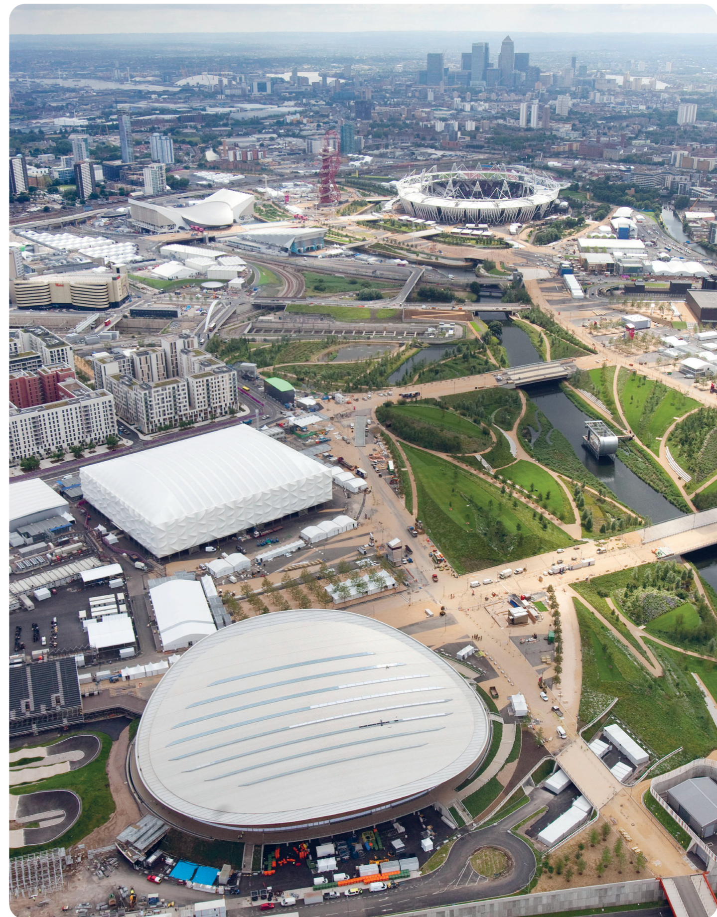
London 2012: aerial shot over Olympic Park.
